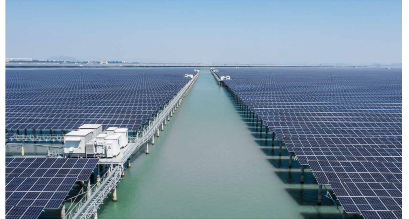
15 Utility Project in the Zhejiang 550MW Watersurface PV Plant
