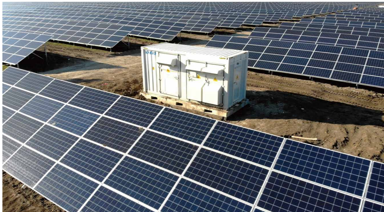
14 Utility Project in the Ukraine 200MW PV Plant
