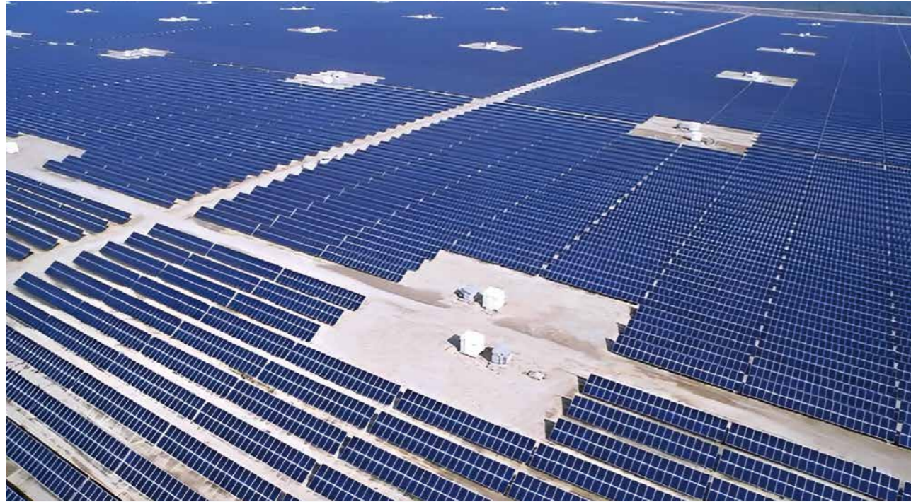
13 Utility Project in the Pakistan 900MW PV Plant
