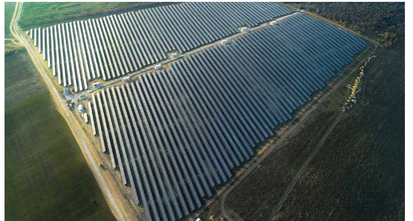
16 Utility Project in the Ukraine 15MW PV Plant
