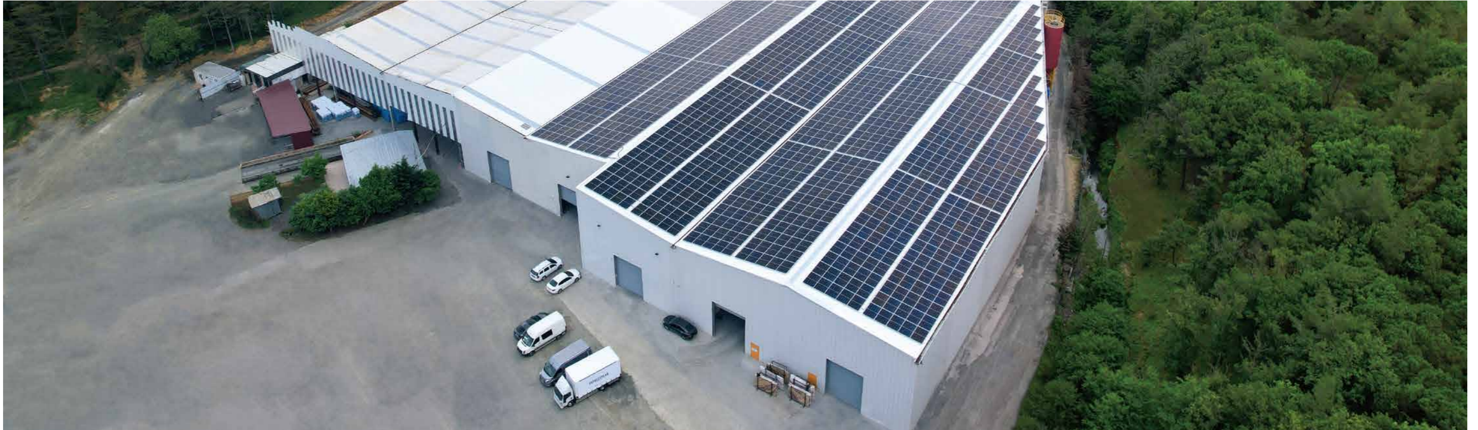
12 Energy cost reduction for Mineral water factory Turkey, 900kW KSG-120CL-M0
